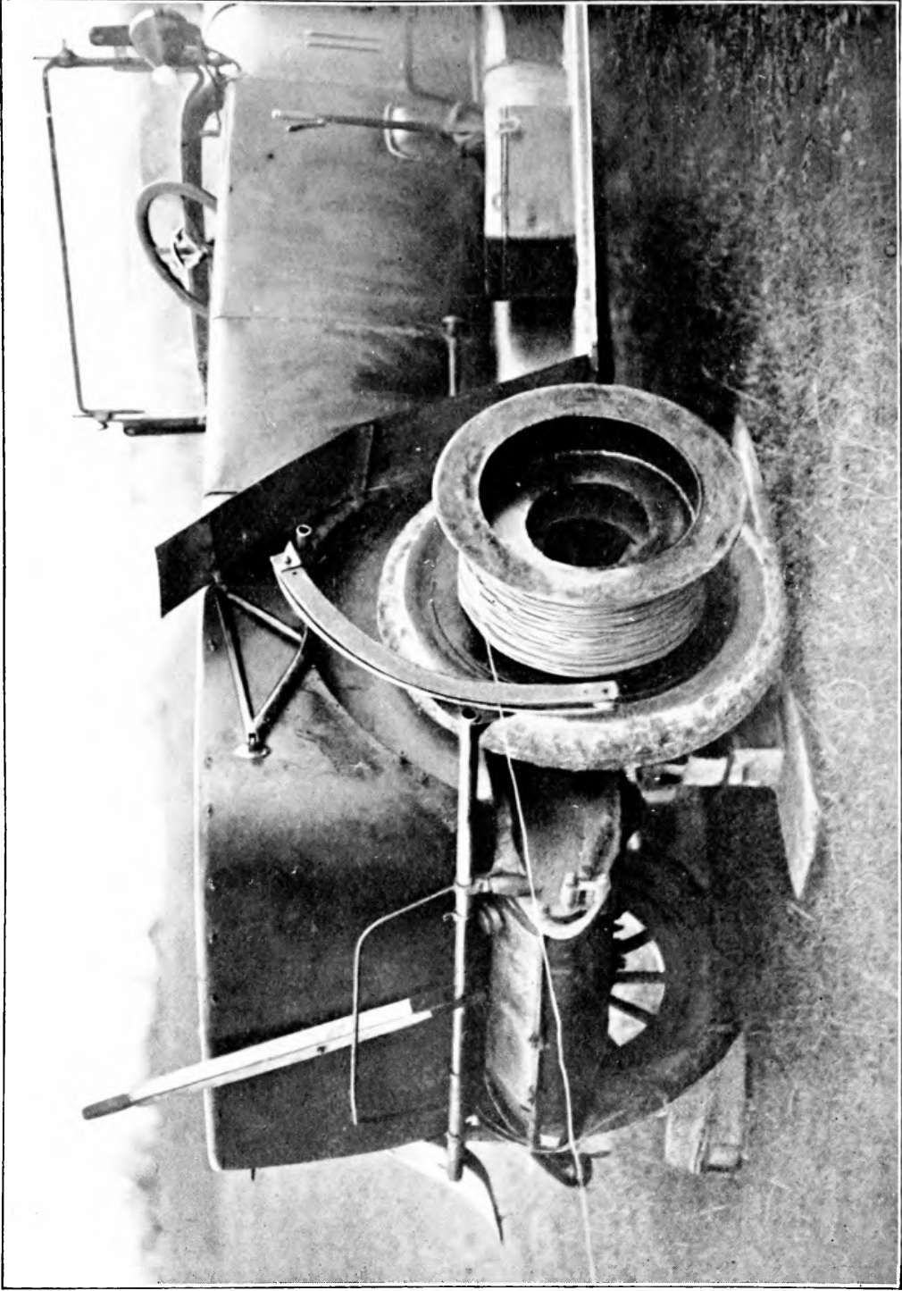
66. A STATIONARY MOTOR-WINDLASS
