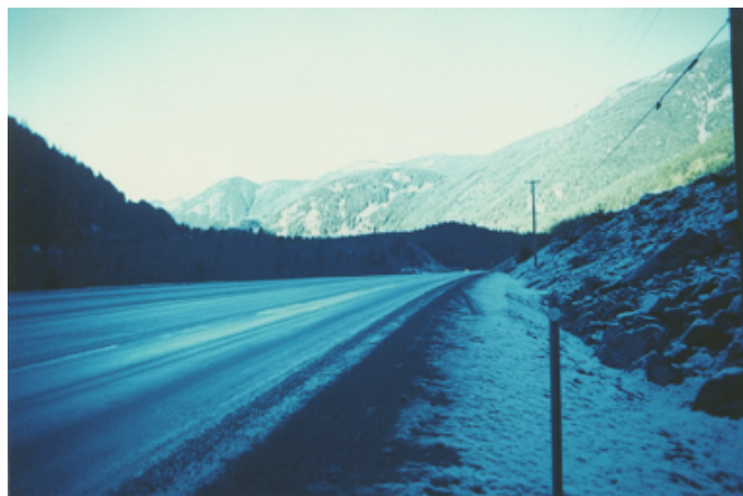
26. Hope-Princeton Highway, Same View - 360 deg. Of mountainous Terrain
